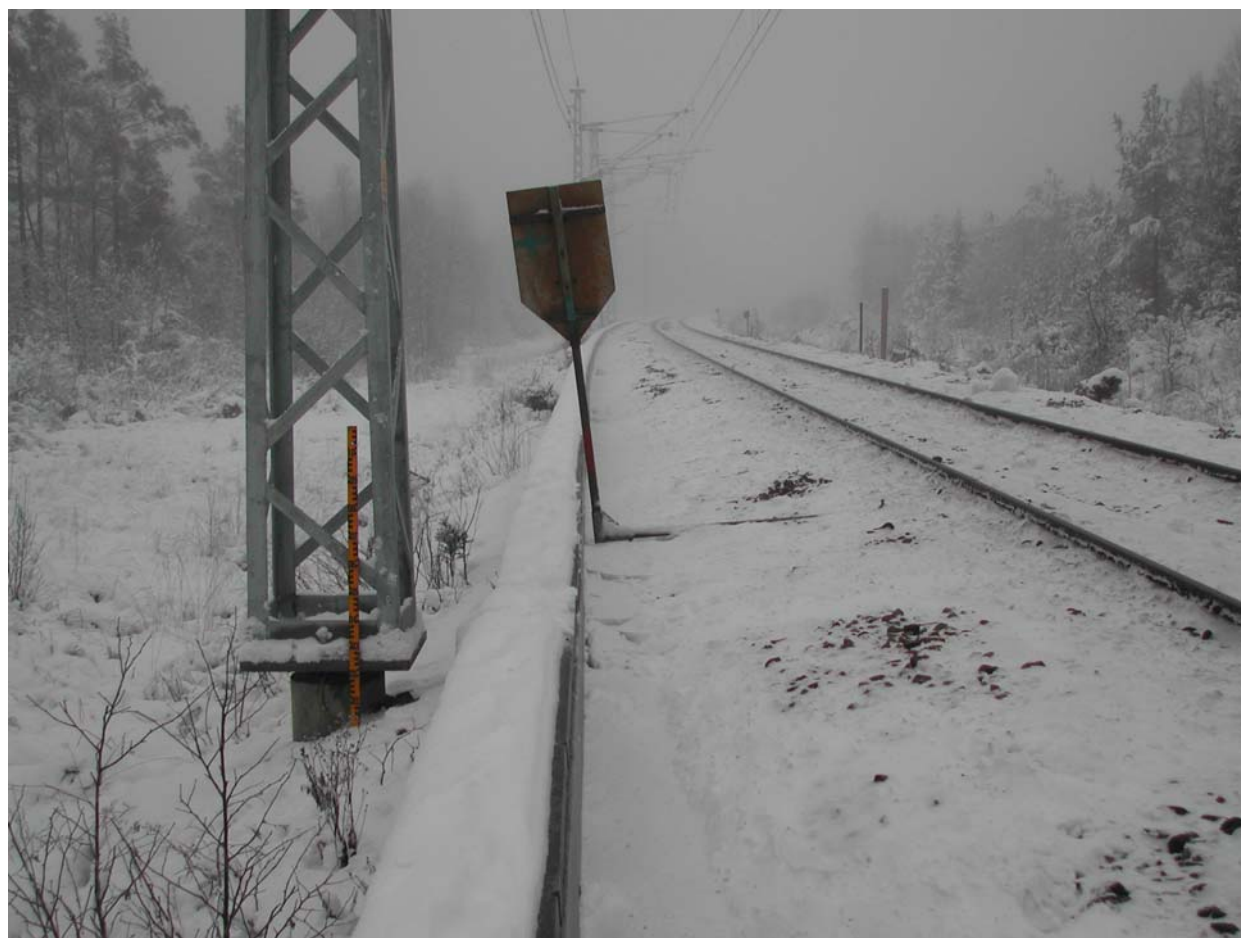
Figur 8-9 Mastfundament 151-16. Opprasing 25 cm
